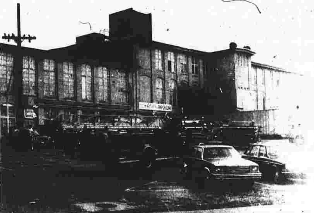
Firefighters responded to a box alarm Tuesday at 240 Pine St. Workers on the main floor of what once was the King's Department Store damaged a water pipe which set off the alarm system. Officials called the damage minor. (Herald photo by Kearns)
